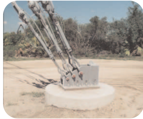
Caissons at Guy Anchor Points
