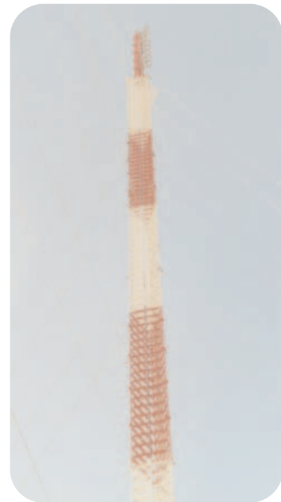
Completed Tower with Lambda Mounting and SHPX FM Antennas
