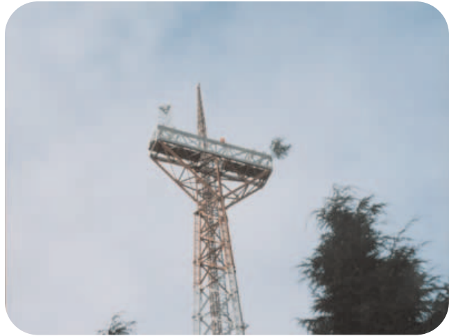
T-Top During Construction
